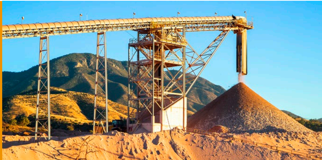
Stockpile, Milpillas mine
