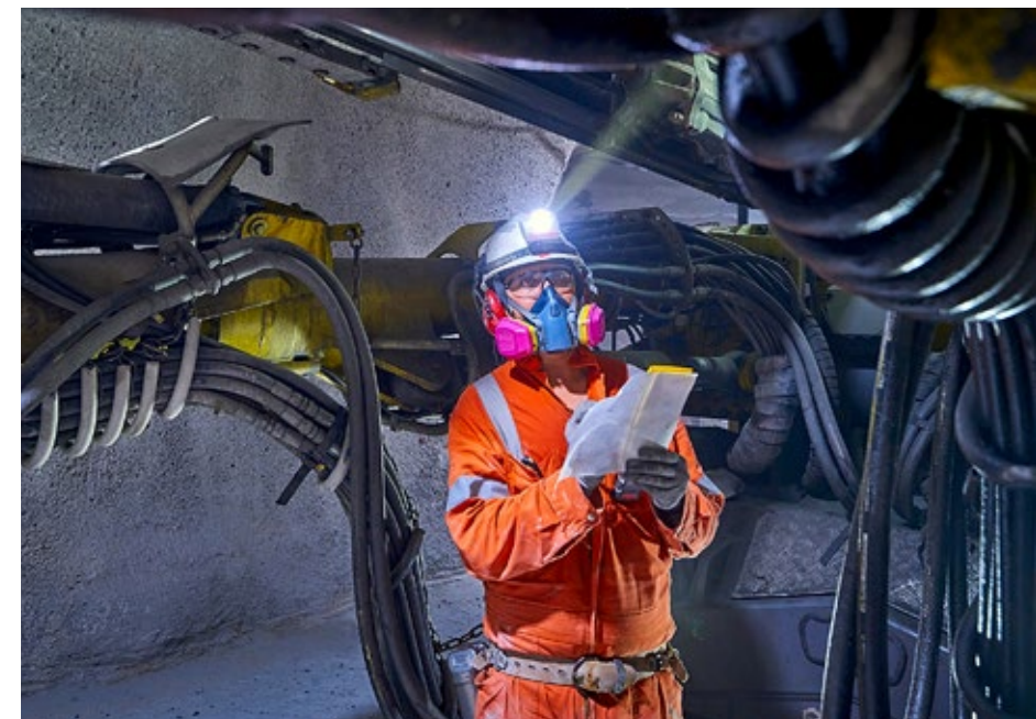
Supervising drill jumbos, Capela unit
