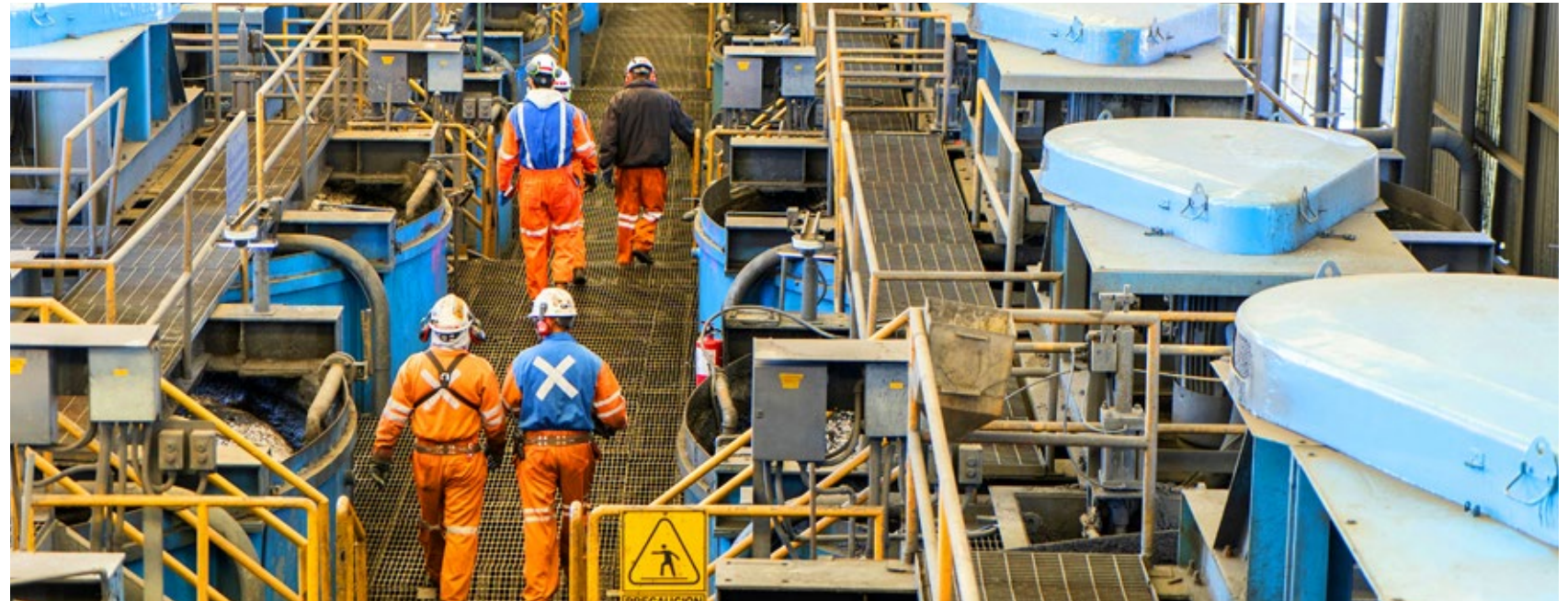
Flotation area at Madero unit
