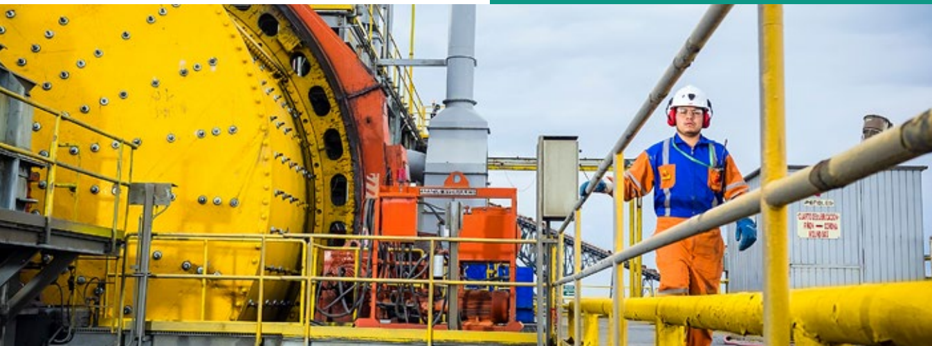
Grinding unit, Madero plant
