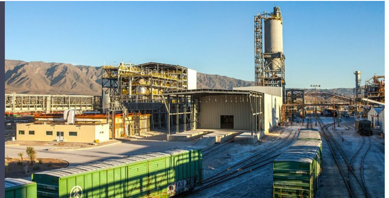
Transport yard at Química del Rey
