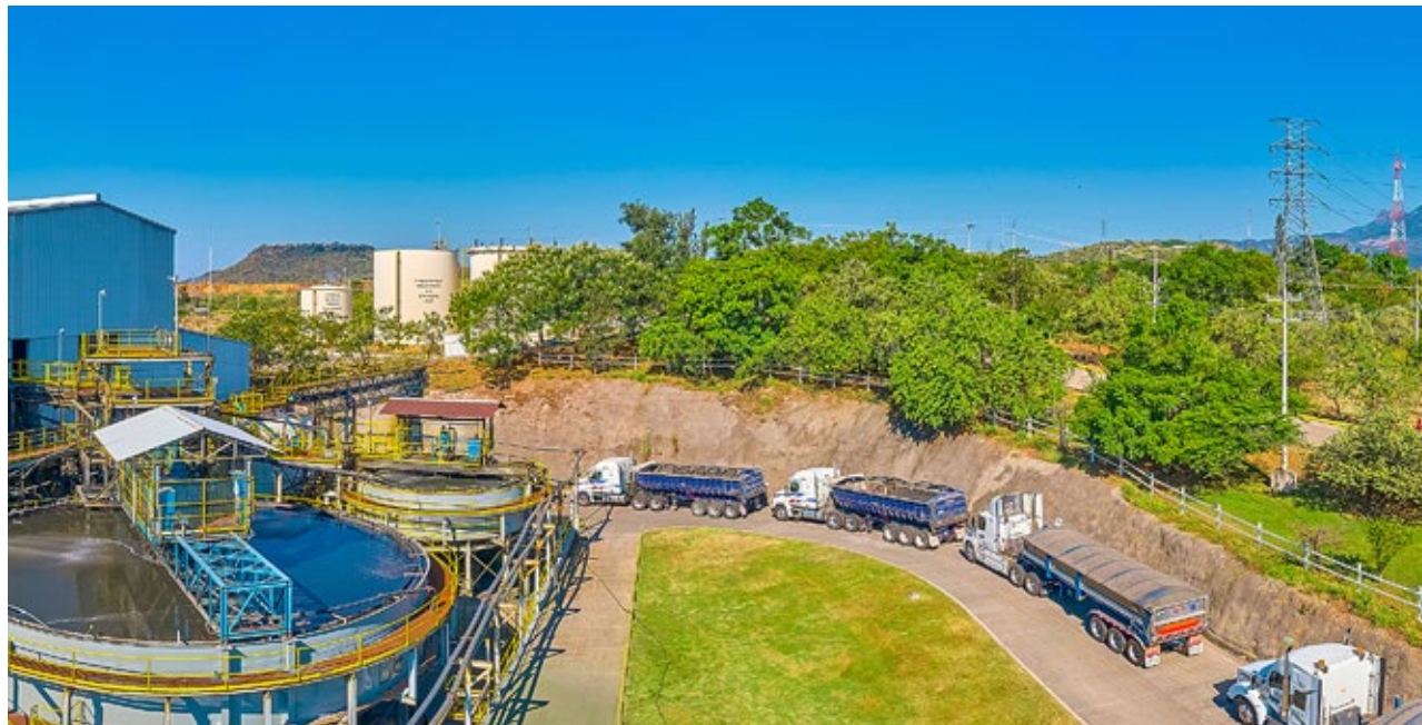
Aerial view of loading area at Tizapa
