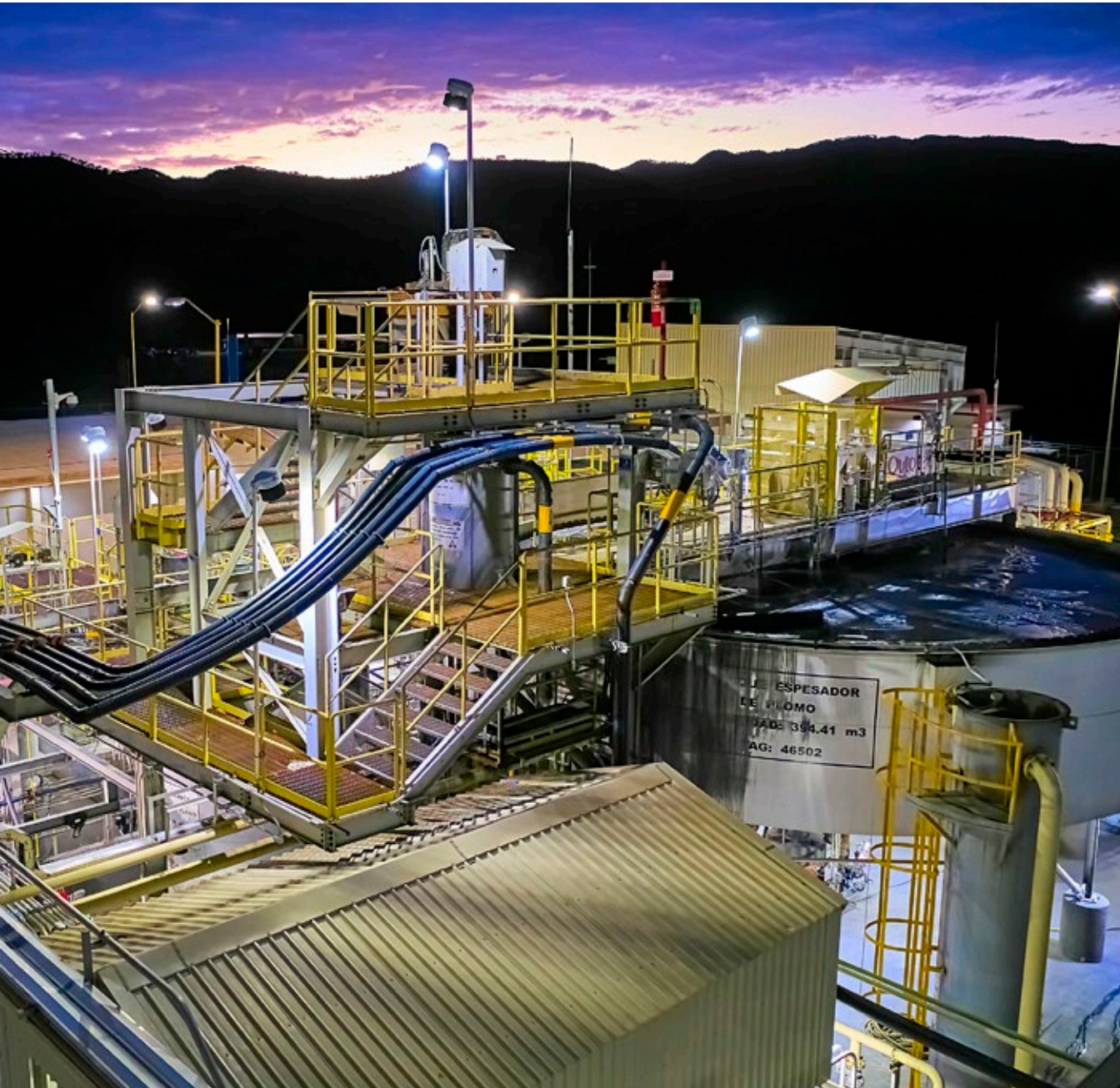
Aerial view at sunset, Capela unit
