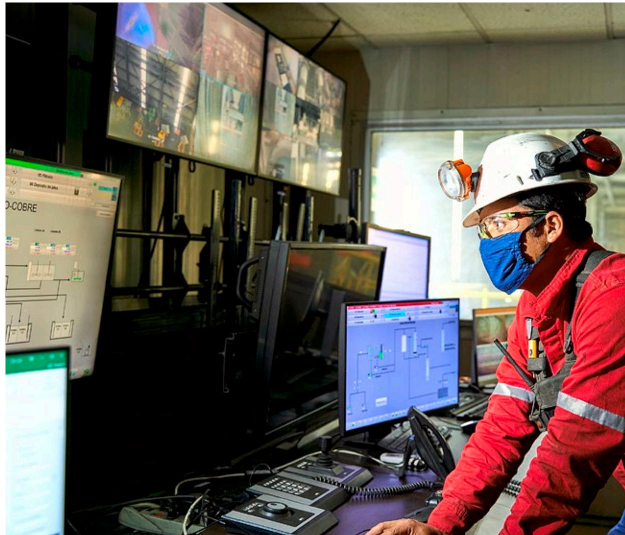
Control room, Tizapa plant
